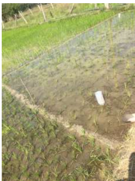
Fig 3. installed perforated pipe for measurement of field water level
